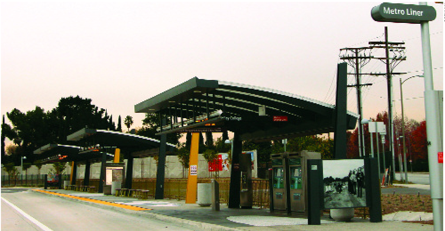
An example of one of the new Metro Liner bus stops in Los Angeles which offers an excellent example of a new public transportation system. Its design incorporates safety, efficiency, comfort and aesthetics. The pavilion provides shelter, illumination, route map, automatic ticket machine, computerized display screen indicating the arrival of next bus, audio announcement system, seating, public telephone and several trash cans.
